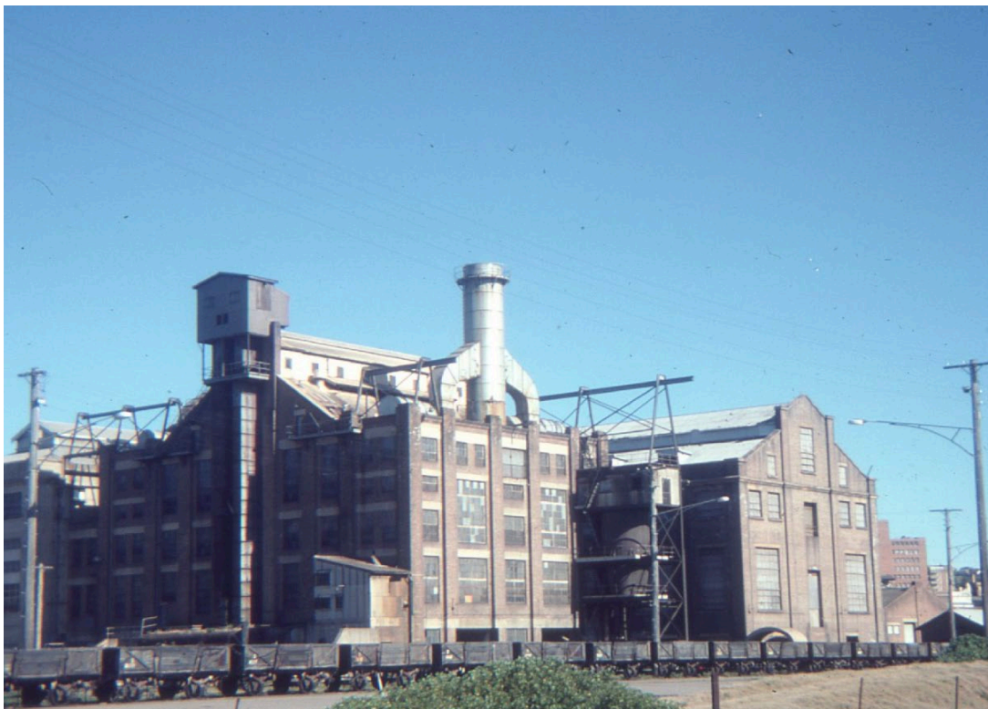
Zaara Street Power Station
