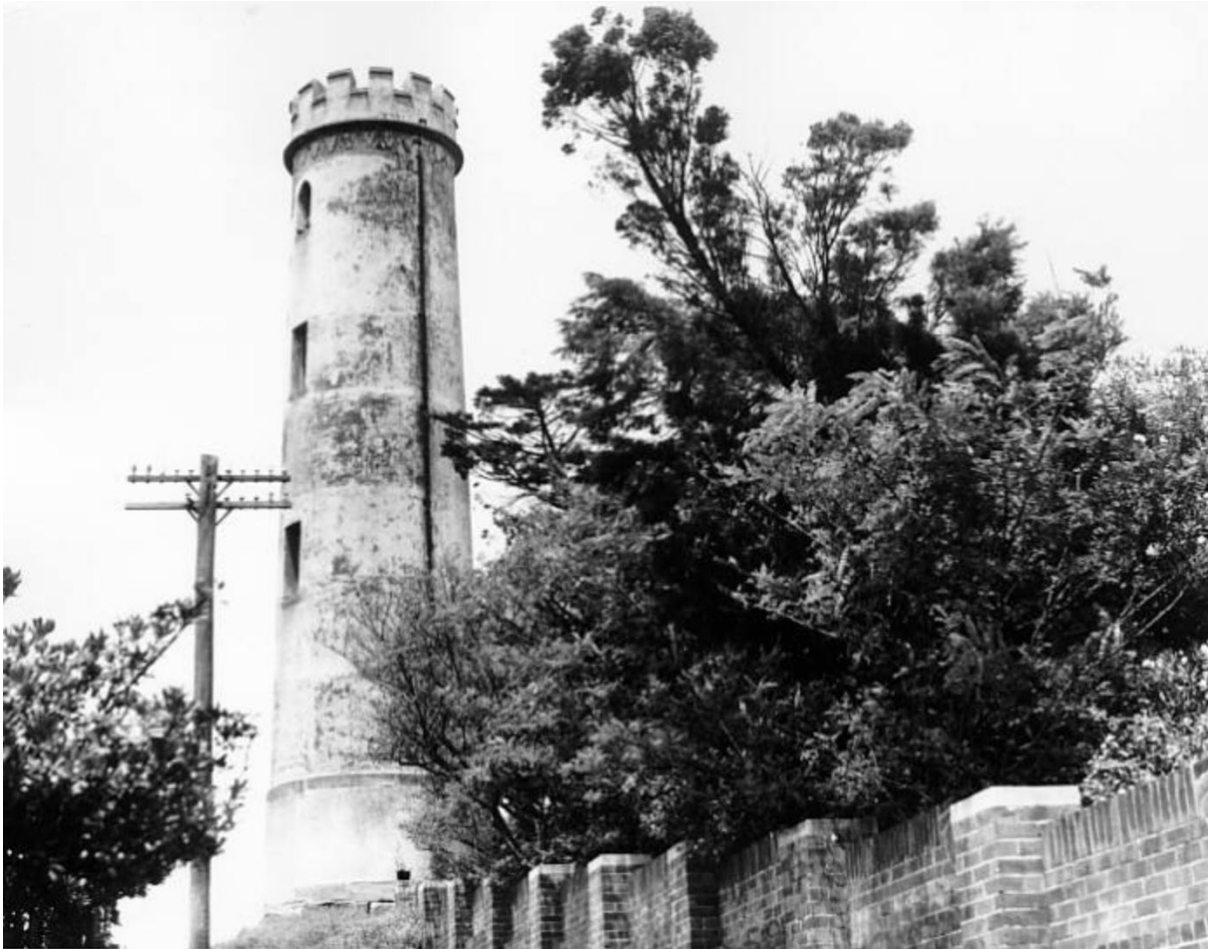
Lead Light Tower
