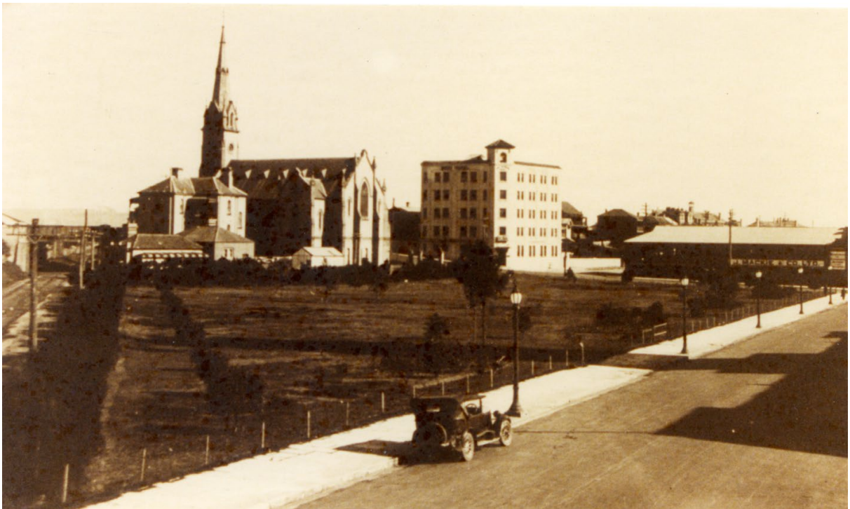
View of Civic Park and adjacent Railway Line
